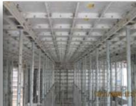
Full aluminum system formwork at Martin Place Residences
