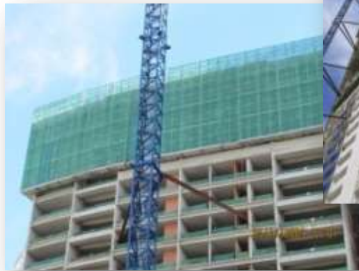
Intelligent computerized self-climbing platform at Martin Place Residences
