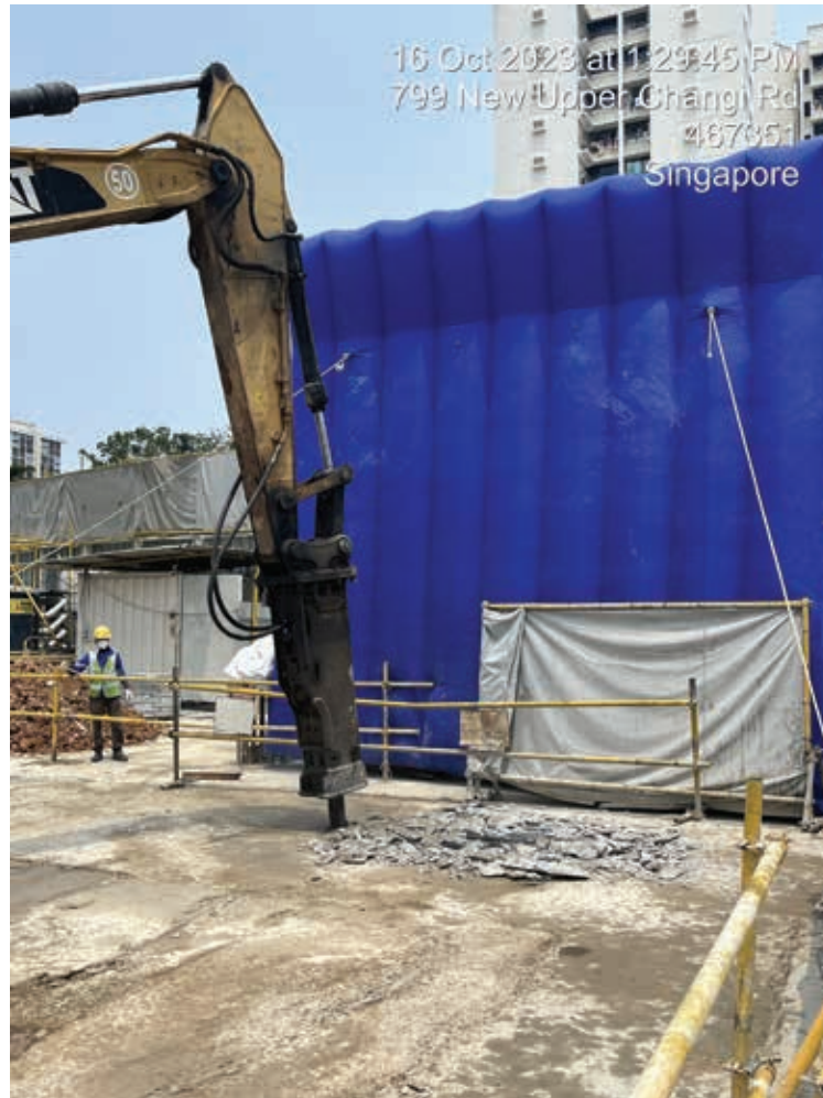
Inflatable Noise Barrier allows for optimum noise reduction and noise mitigation solution erected on site
