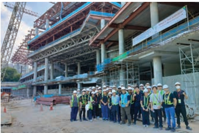
ITE trainees visited Punggol Regional Sports Centre worksite on 2 August 2023 to study DfMA design and implementation.
