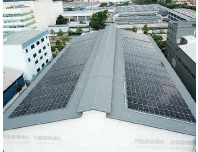
Solar panels installed on West facing roof of Chin Bee Factory, West and East facing roofs, covering a total area of 4,008 m 2 . Solar panels will supply 6.1 million kWh of solar energy to Chin Bee Factory in the next 12 years.
